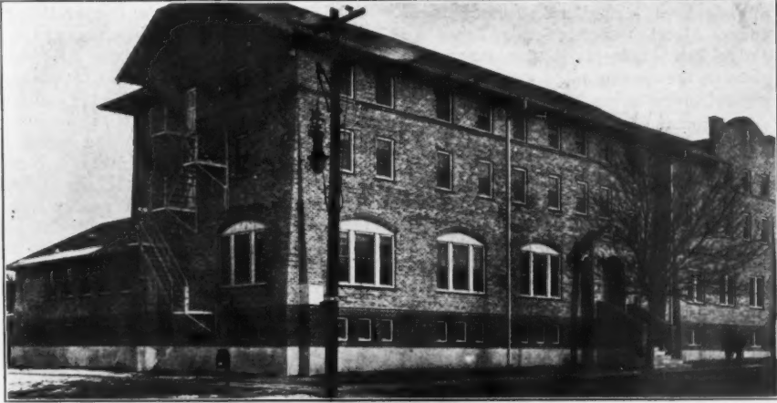
THE GLENARM BRANCH OF THE Y. M. C. A., DENVER
